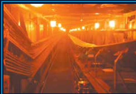
▲ BF Flux Conveyor System
