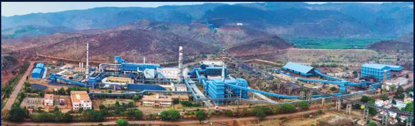
▲ 1.2 MTPA Total Pallet Plant
